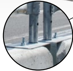
PANEL SECURED TO THE CONCRETE BARRIER WITH BOLTS
